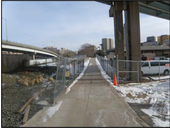
Interim Route of the East Coast Greenway behind the State Armory
