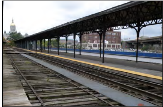
Existing Center Platform at Hartford Union Station
